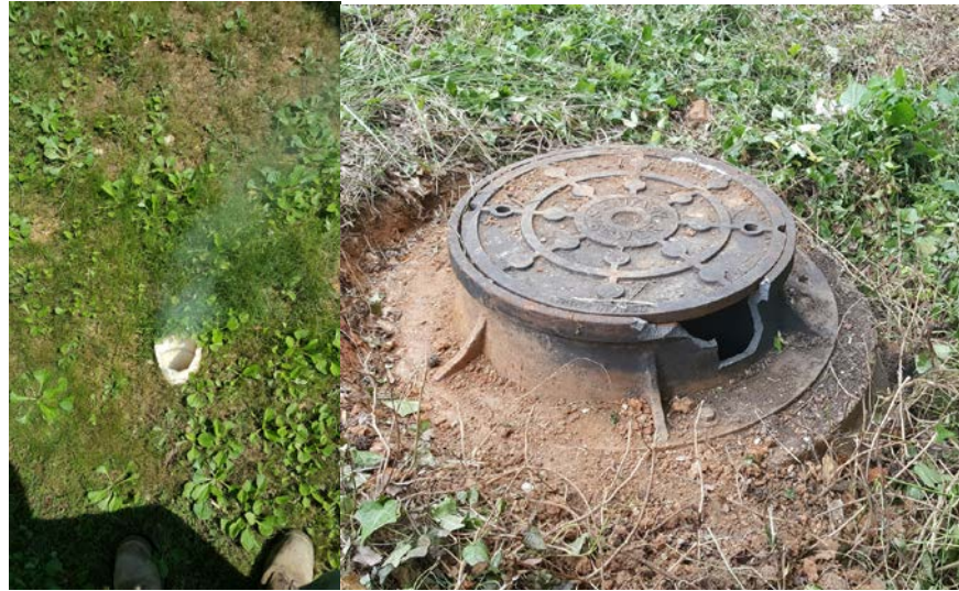
Figure 13: Damaged Cleanout Cap and Manhole Ring
